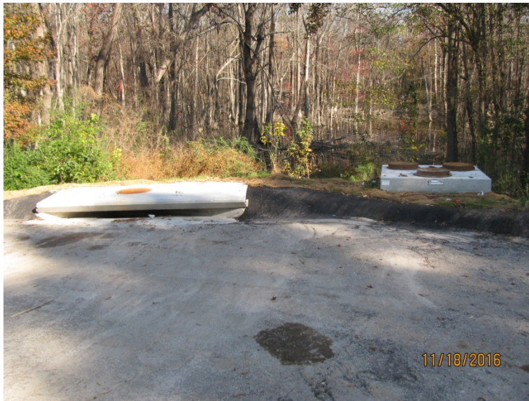
Surface view of Site 3 MTD and inlet
