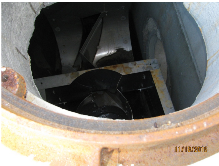
Interior view of Site 3 MTD
