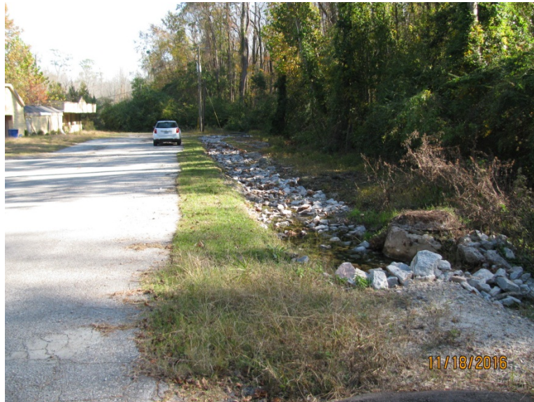
Upstream side of the swale at Site 5
