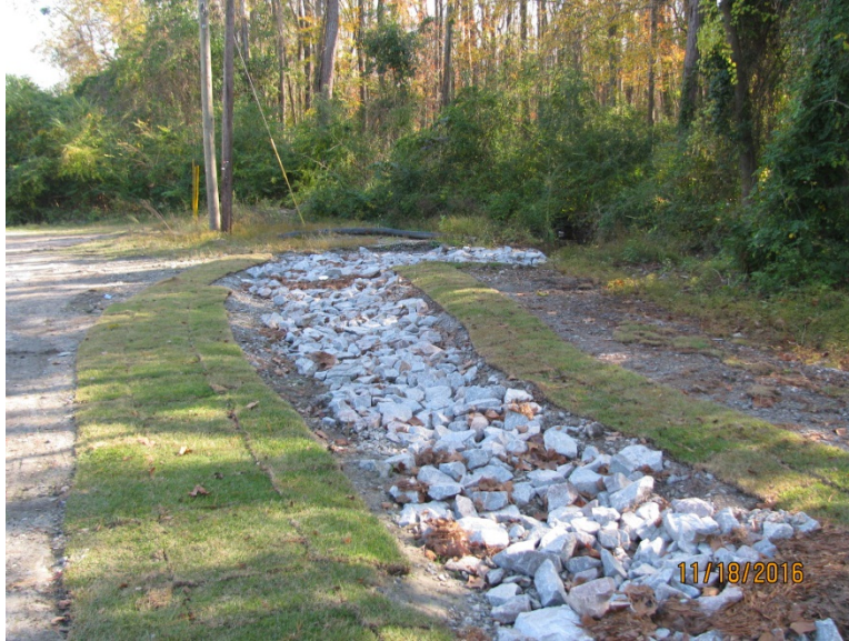
Downstream side of the swale at Site 5
